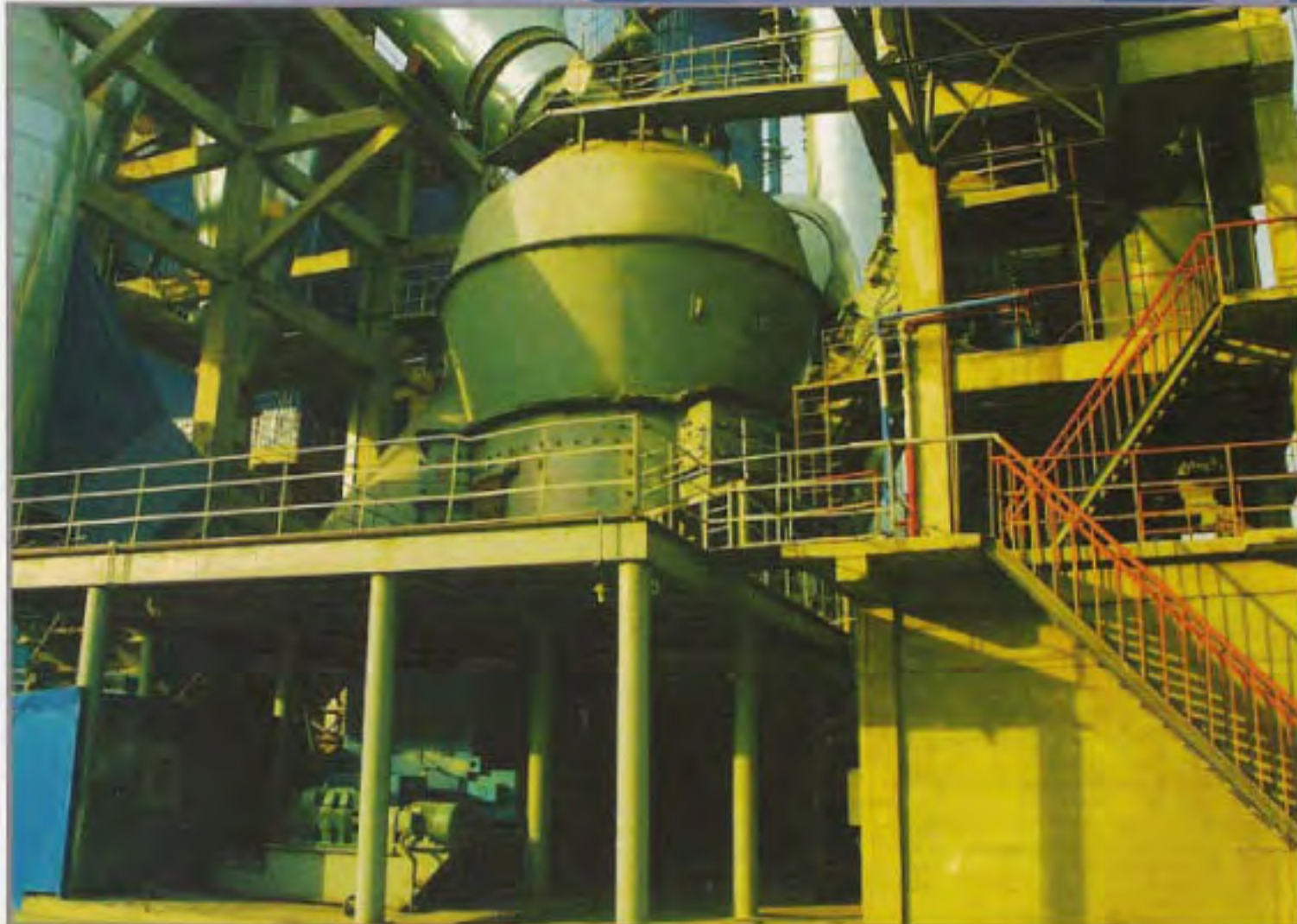
日产3000吨水泥生产线立式生料磨 Vertical raw mill for 3000tpd cement production line
