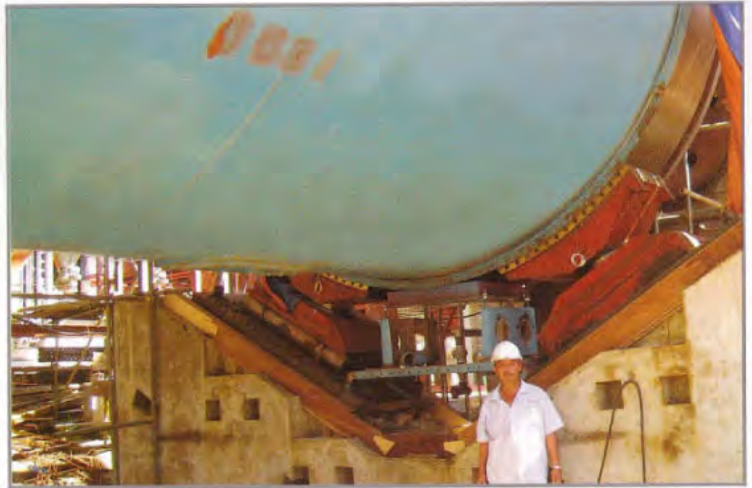
菲律宾Φ5m原料磨安装中 Φ5m raw mill under assembly in Philippines
